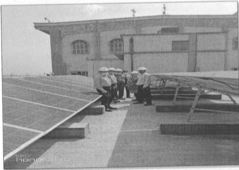
Solar PV Plant at Service Building
